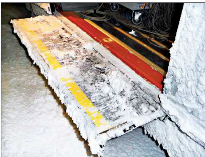
Photos 7: Movable door step with snow and ice build-up on a step.
