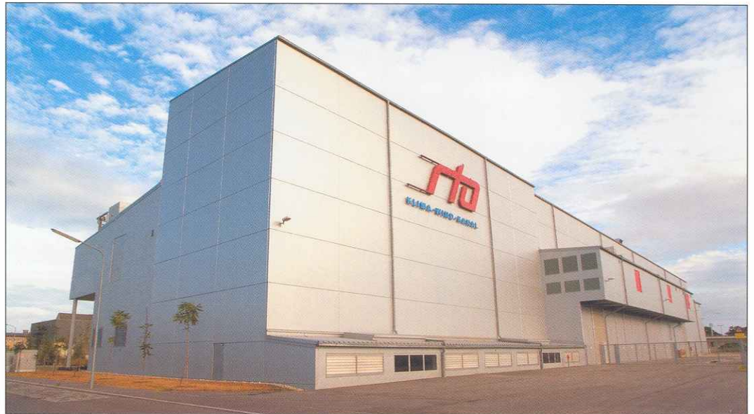
The main building of RTA, containing two climatic wind tunnels, two preparation halls, the cooling plant and the power converter units.
