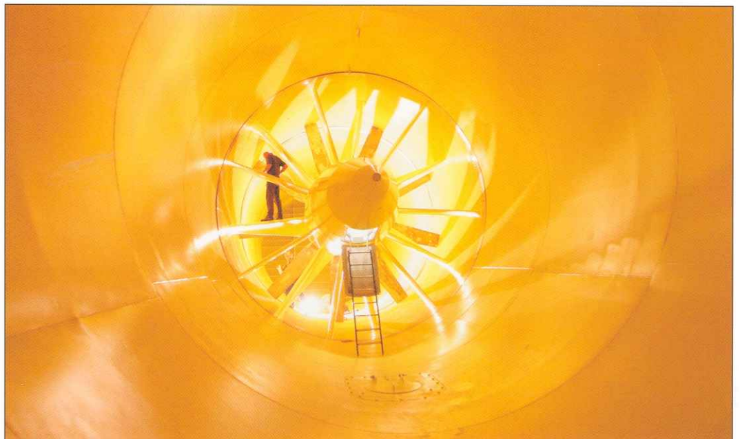
Maintenance work in the 0.5 MW fan for the small CWT.
